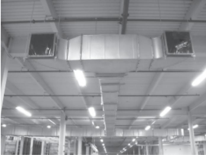
Several months back Don Park USA from Conley, Georgia and Action Electrical & Mechanical Contractors from Smyrna, Georgia teamed up to take on the fabrication and installation of duct work for the Paint Facility at the new Kia plant in West Point, Georgia. In less than 5 months 240,000 pounds of aluminized steel duct work and fittings were manufactured and delivered by Don Park USA and installed in the plant by Action Electric & Mechanical Contractors.
